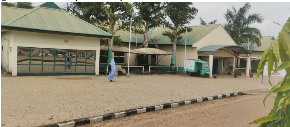
Plate I: Exterior view of KASU Library Source: Field survey (2025).
