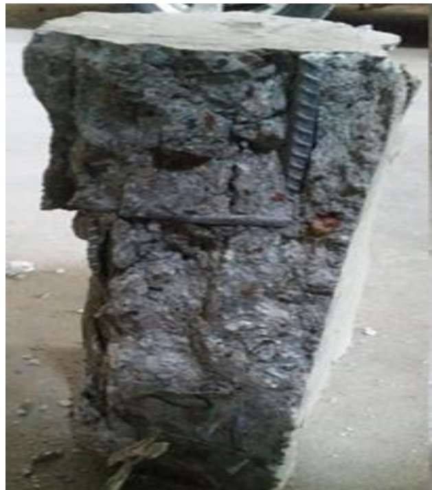
Figure 3.0: Typical Failure mode of Control specimens
