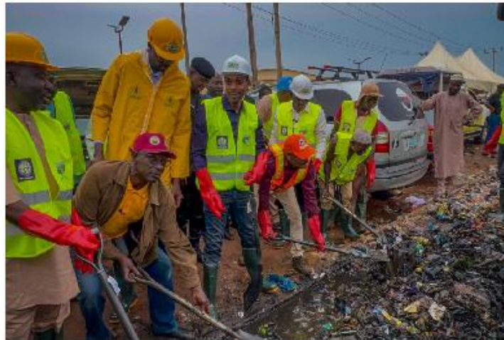
Plate II: Kaduna State Government official clearing drainage
