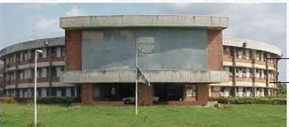
Plate III: The use of both vertical and horizontal shading Source: Author`s fieldwork (2025).
