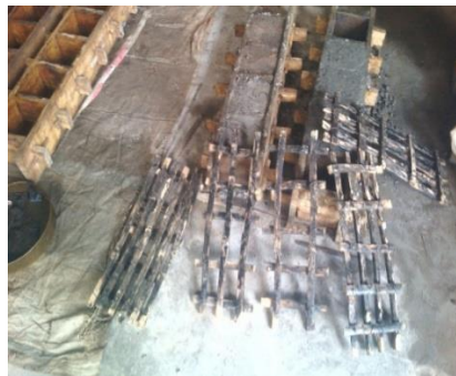
Plate 1: Some of the prepared Bamboo reinforcement
