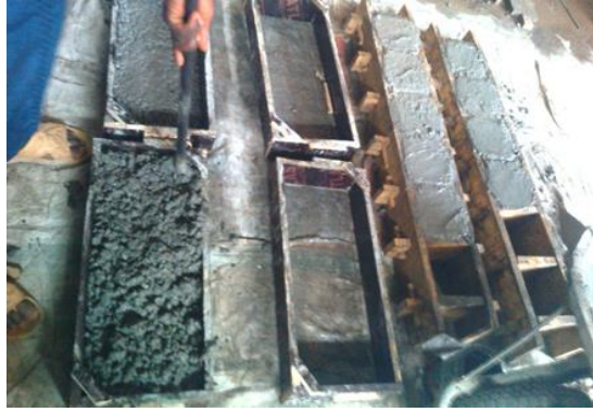
Plate 2: Casting of the slab specimens
